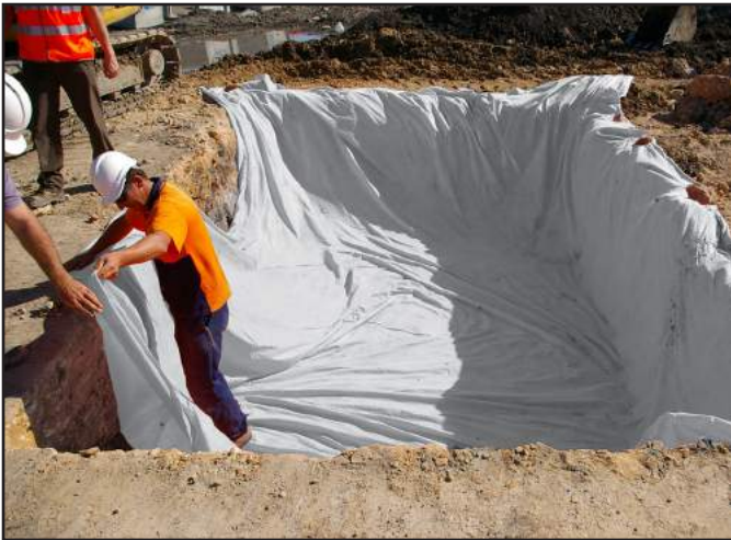
Step 3 - Lay geotextile.
